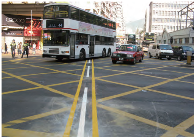
Road marking works at Argyle Street, Mongkok.
