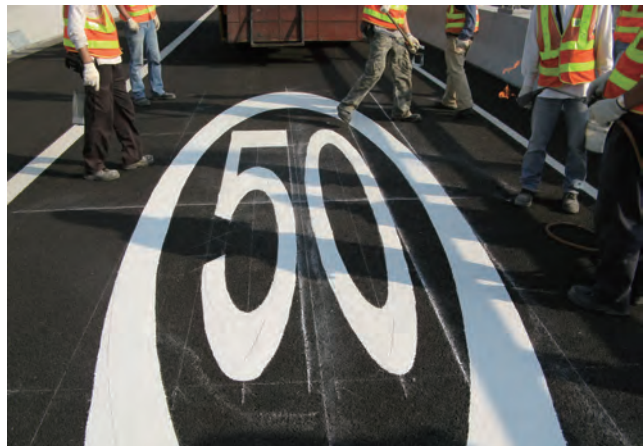
Road marking works on a major bridge deck.
